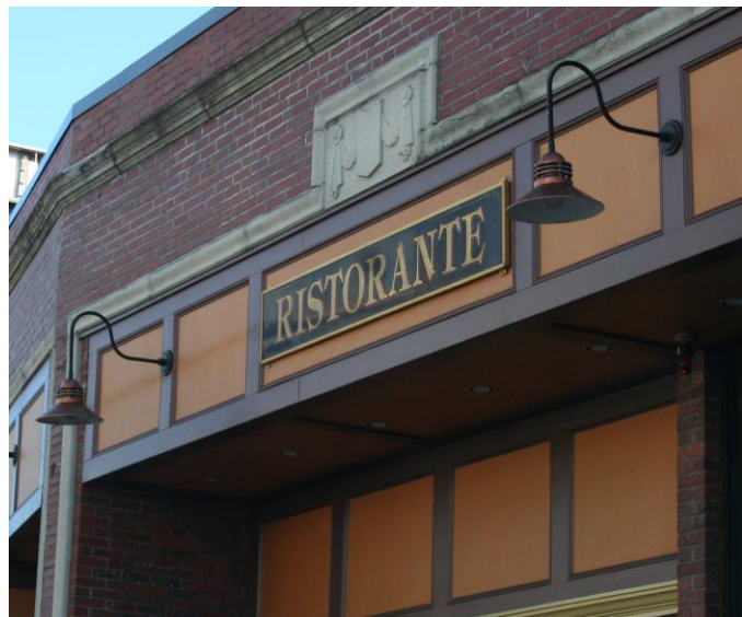
Figure 3-7: Hangover Lights Illuminating Il Capriccio's Sign
