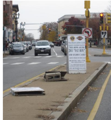
Figure 4-30: Weather Related Instability of A-Frames
