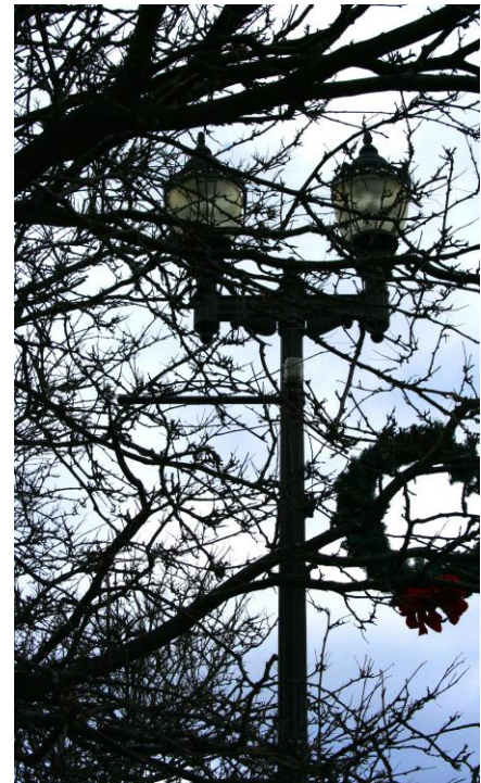
Figure 3-11: Light Post Blocked by Tree Branches
