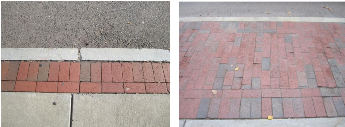
Figure 3-27: Brick Accents in Sidewalk in Downtown Watertown
